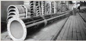
**1933** Expanding on earlier research in the process of fusing glass to steel, A. O. Smith introduces the first large, single-piece glass-lined brewery tank. Over the next 32 years, the Company produced more than 11,000 glass-lined brewery tanks.
